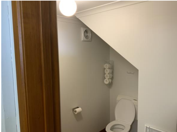
Figure 3 and Figure 4 – Water Closet located under stair does not achieve ceiling height of at least 1.2m
